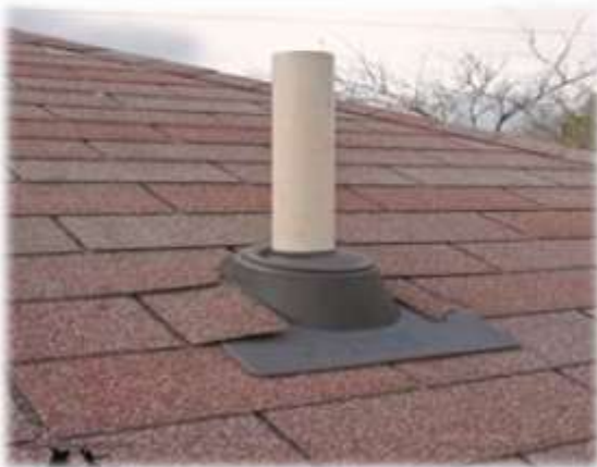
Rooftop Vent Pipe
